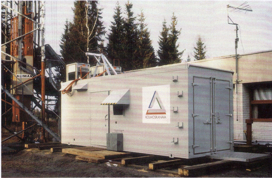
FIG 1 40-kW TV container at site in Finland. Dimensions without external fittings (L x W x H): 7 m x 2.5 m x 2.7 m
