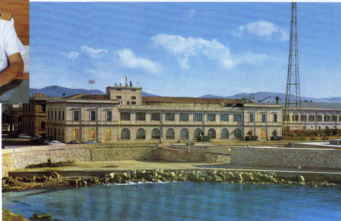
FIG 1 Mariteleradar, the Institute for Telecommunications and Electronics of the Italian Navy, was established in Livorno in 1916 by Admiral G. Vallauri. The institute is involved in technical and scientific activities, mainly in the following fields: EMC, antenna systems, telecommunications, radar, electronic warfare, infrared. The first Italian radar system was developed by Mariteleradar.
